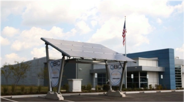
Solar Array with Integrated EV Charging
