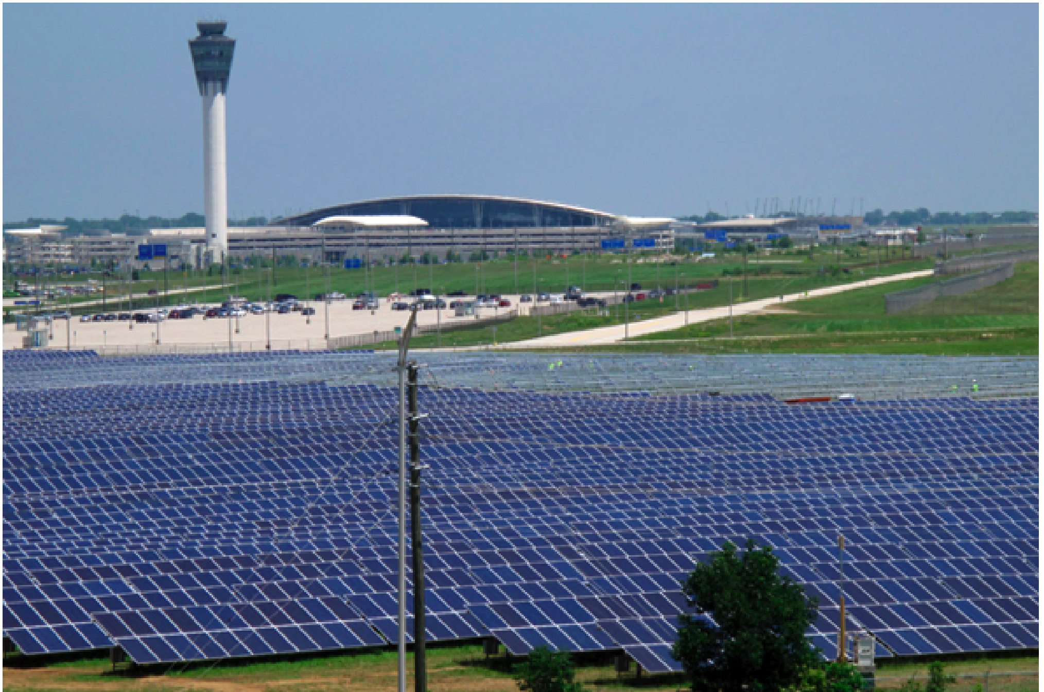
Indianapolis Airport solar farm
