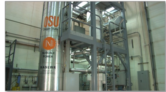
One-third scale Test Facility
